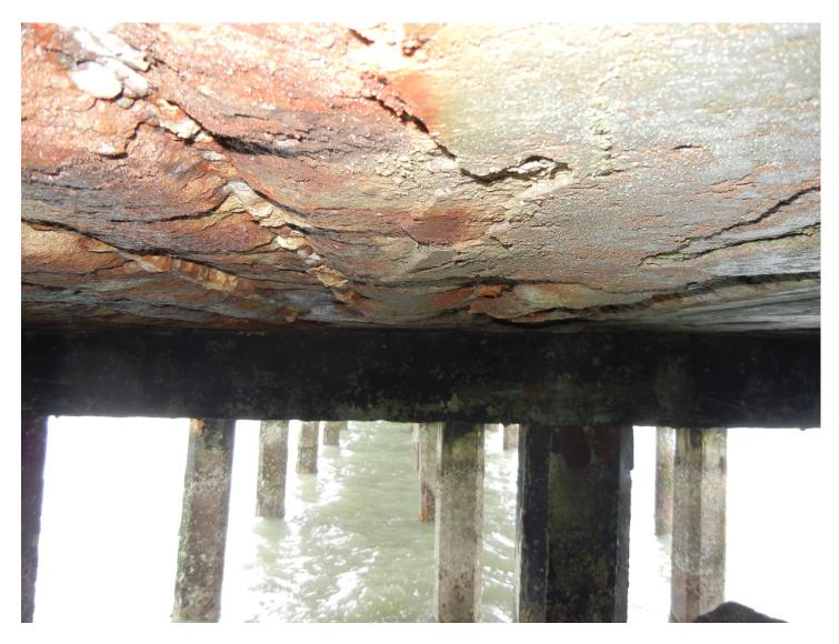
Image 14: On the underside of the concrete deck surface of the Pier, the bottom layer of concrete has spalled off, exposing the structural rebar, which has snapped and failed for the most part, throughout the entire length of the 3,000 foot Pier. On the upper right, see the partially remaining layer of concrete that was applied to the underside in 1984, to prolong the life of the structural rebar. (Photo Credit: Roger Miller)
